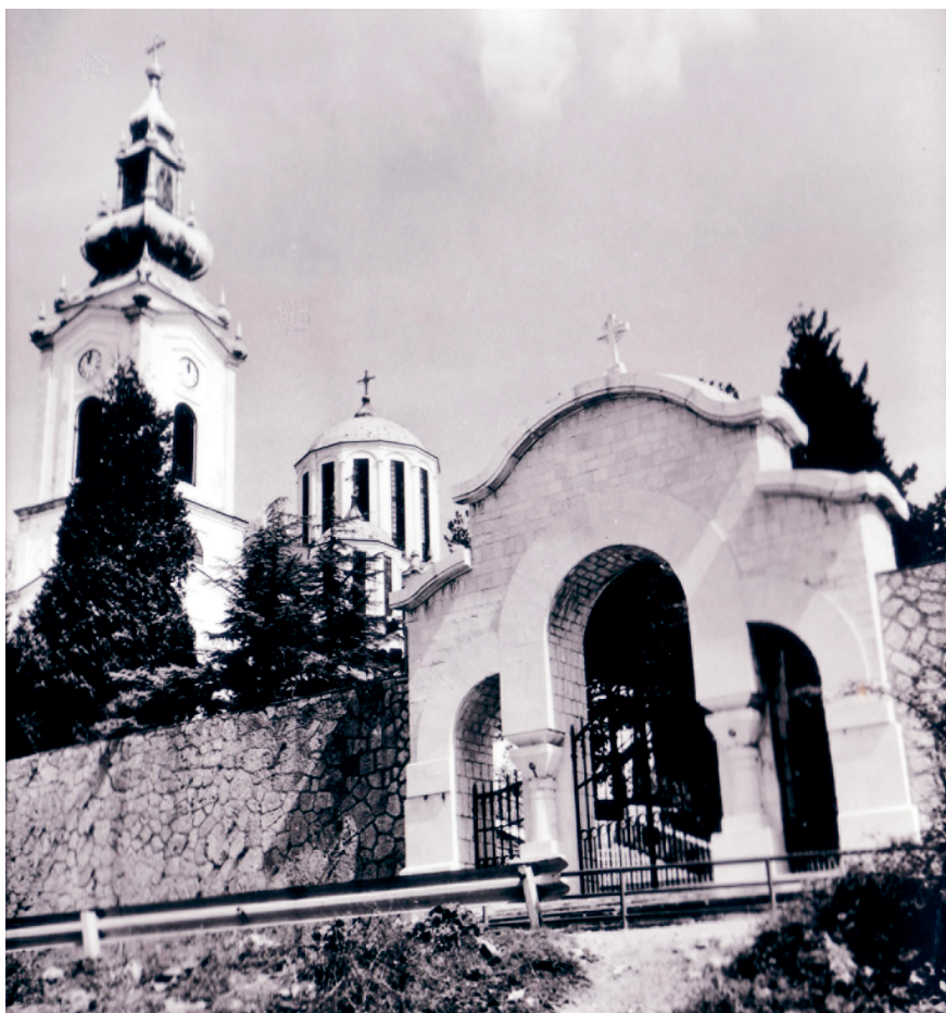
Figure 3. Entrance gate, project by Momir Korunović, a photo taken by Ćiril Ćiro Raić
